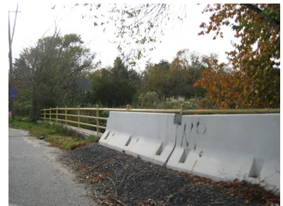
Railing/jersey barrier bridge (-)
