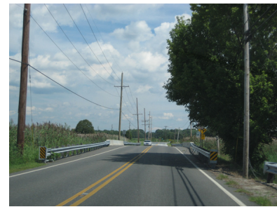
Jersey barrier bridge (-) Narrow road, no shoulders (-/+)
