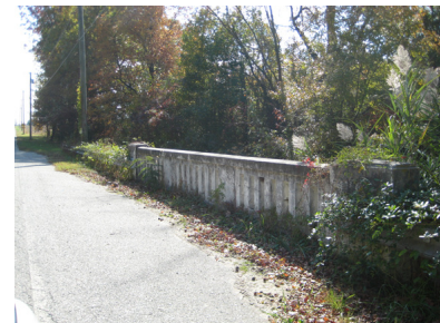
Open parapet bridge (+)
