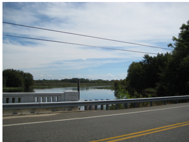
Open parapet bridges (+)
