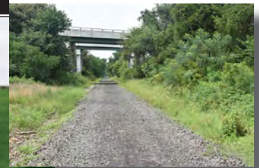
Figure 66 DelDOT's preferred concept utilizes the existing bridge parapet and bridge columns without modification. The rail-trail, relocated to the outside of the existing columns, will require a low retaining wall
