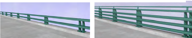
Figure 84 Example of CalTrans Rail Type 10 (left) and 20 (at bicycle pedestrian height of 54") approved for use at Test Level 4
