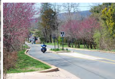
12' splitter with gore area pavers
