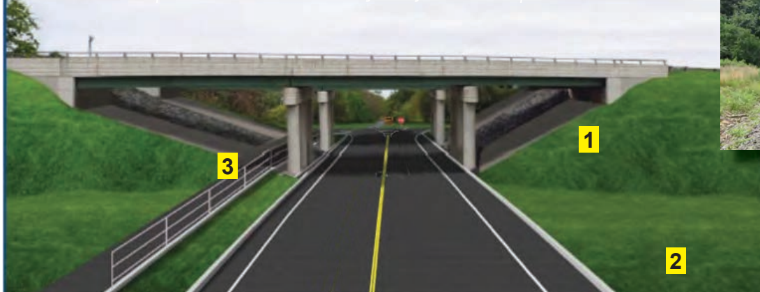
Figure 66 DelDOT's preferred concept utilizes the existing bridge parapet and bridge columns without modification. The rail-trail, relocated to the outside of the existing columns, will require a low retaining wall
