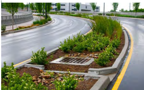
Figure 92 Median bio-swale
