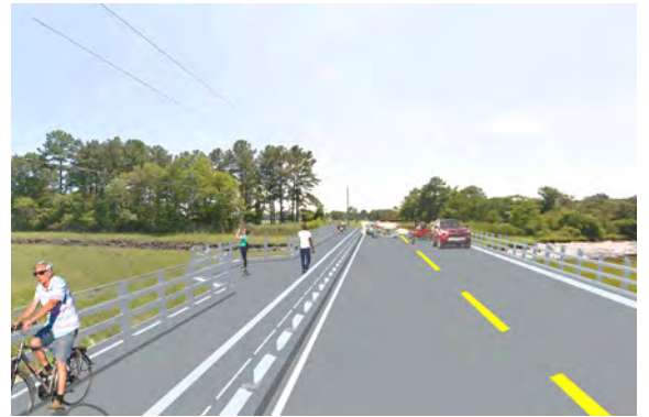
Figure 85 Illustrative concept showing a combined structure used to accommodate both the vehicular travel lanes and the shared use pathway with an overlook to Canary Creek
