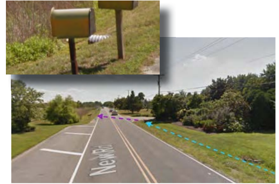
Figure 90 Ditchline on WB side of New Road leading to outlet on EB side (inset)
